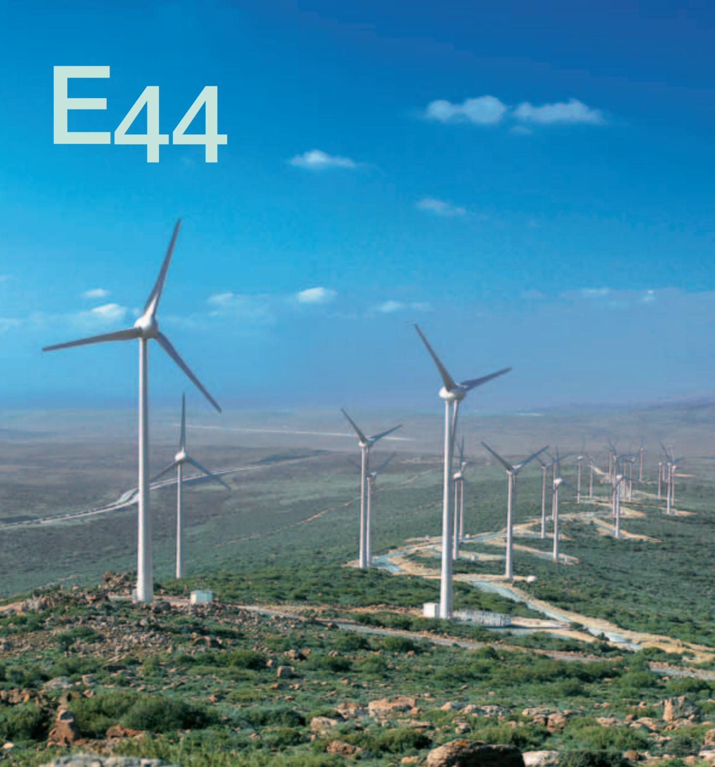
Developed as a strong-wind system for the international market, the E-44 wind turbine sets the benchmark in the medium power range. As all other ENERCON wind turbines, the E-44 is also provided with ENERCON's efficient rotor blade design. With a rated power of 900 kW, maximum use is made of prevailing winds at strong wind sites.
